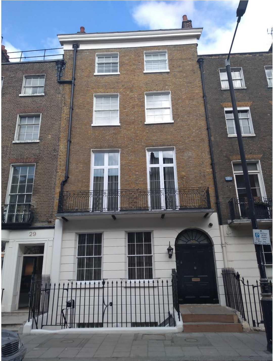
Front elevation, 30 Chapel Street SW1
